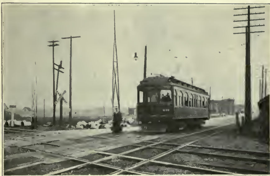
FIG. 250. GRADE CROSSINGS. Chicago & Interurban Railroad crossing of the Chicago, Rock Island & Pacific Railway at 90th Street and Vincennes Road.
